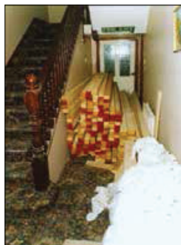
Figure 9: A blocked corridor with incorrect signage
